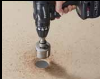
Boor verticaal in planken
